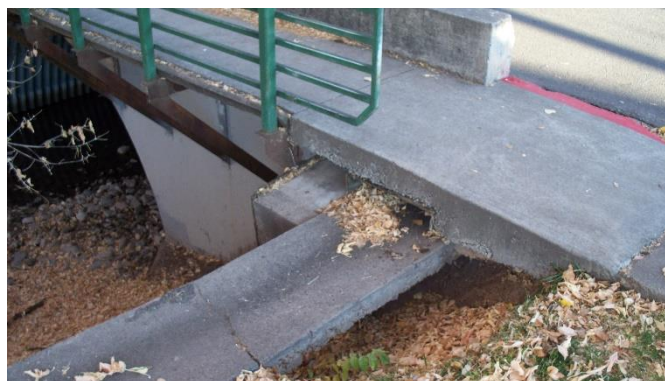
Example of cavity formed at the creek and sidewalk
