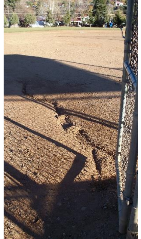
Erosion at dugout entrance
