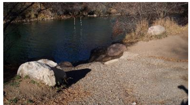
Example of rock armoring of river bank
