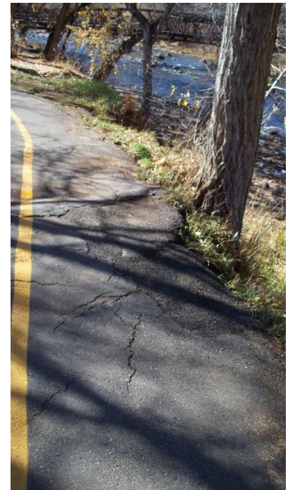
Heaving section of the trail
