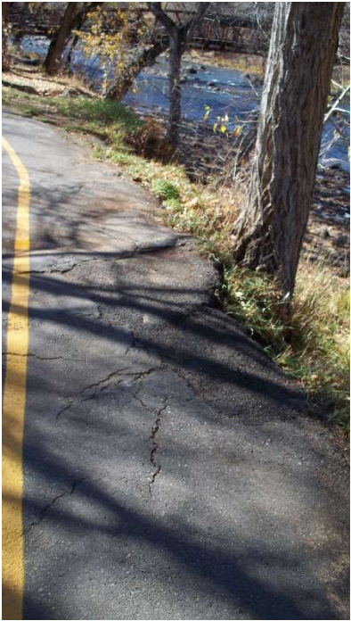
Heaving section of the trail
