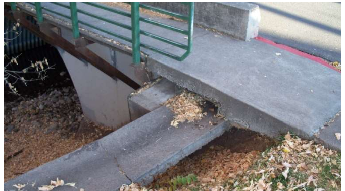
Example of cavity formed at the creek and sidewalk
