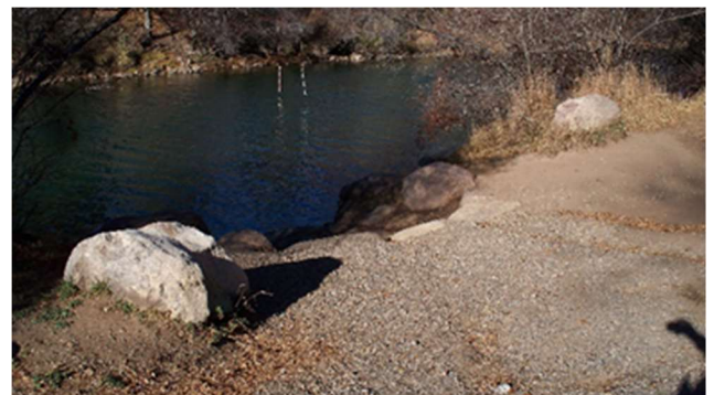
Example of rock armoring of river bank
